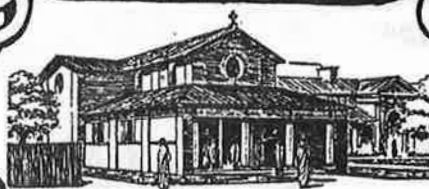
Exterior of the church at St. Michael's
