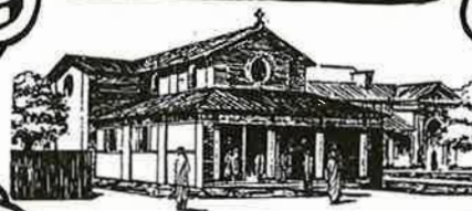
Exterior of the church at Silchester
