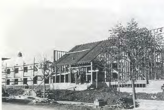
The church under construction in early 1954
